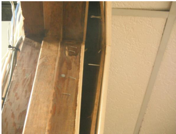
Wall Sheathing Separation 1
