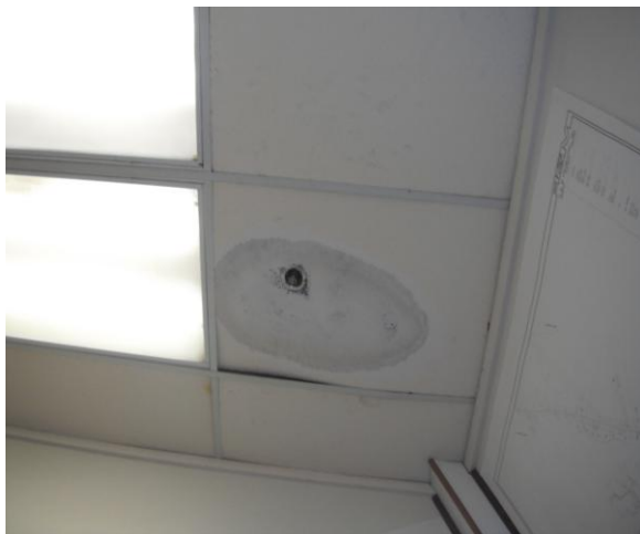
Ceiling Water Damage 1
