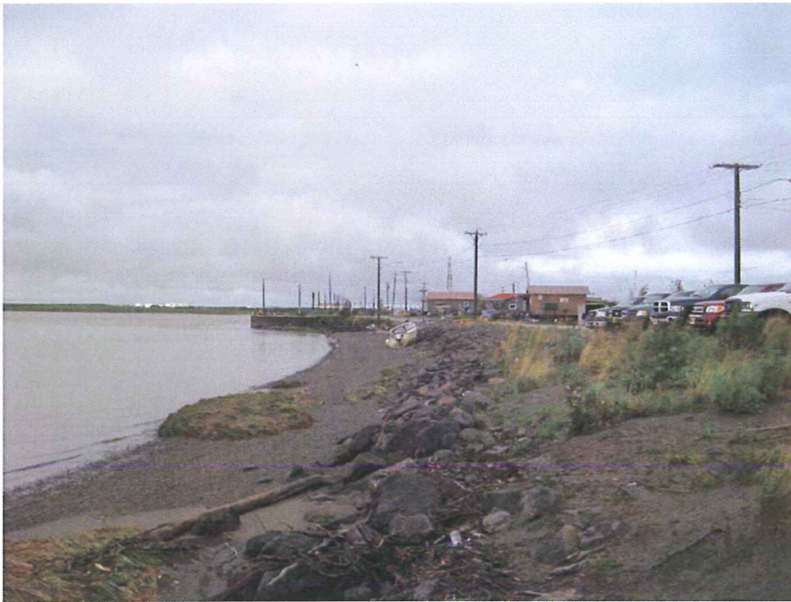
Photo 9. Entrance channel town side bank with “B” rock slope protection.
