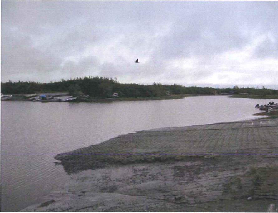
Photo 8. South launch ramp articulated concrete block section.
