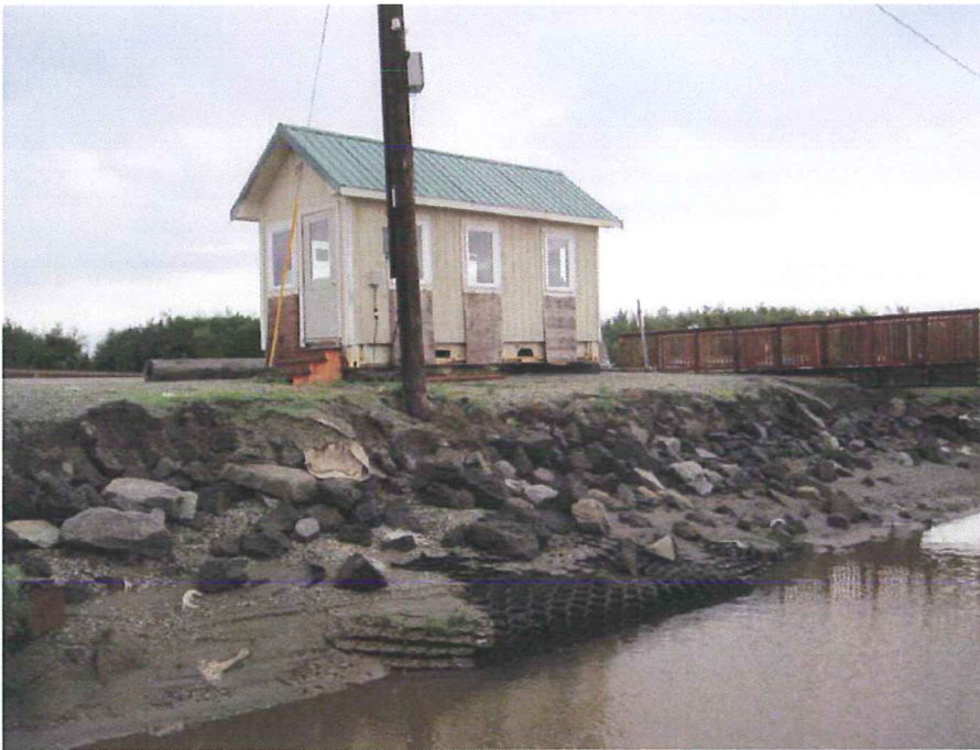
Photo 4. North bank "B" rock and exposed geoweb.
