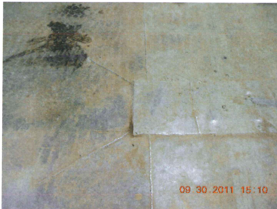
Various welded metal patches on floor to stem the cracks.
