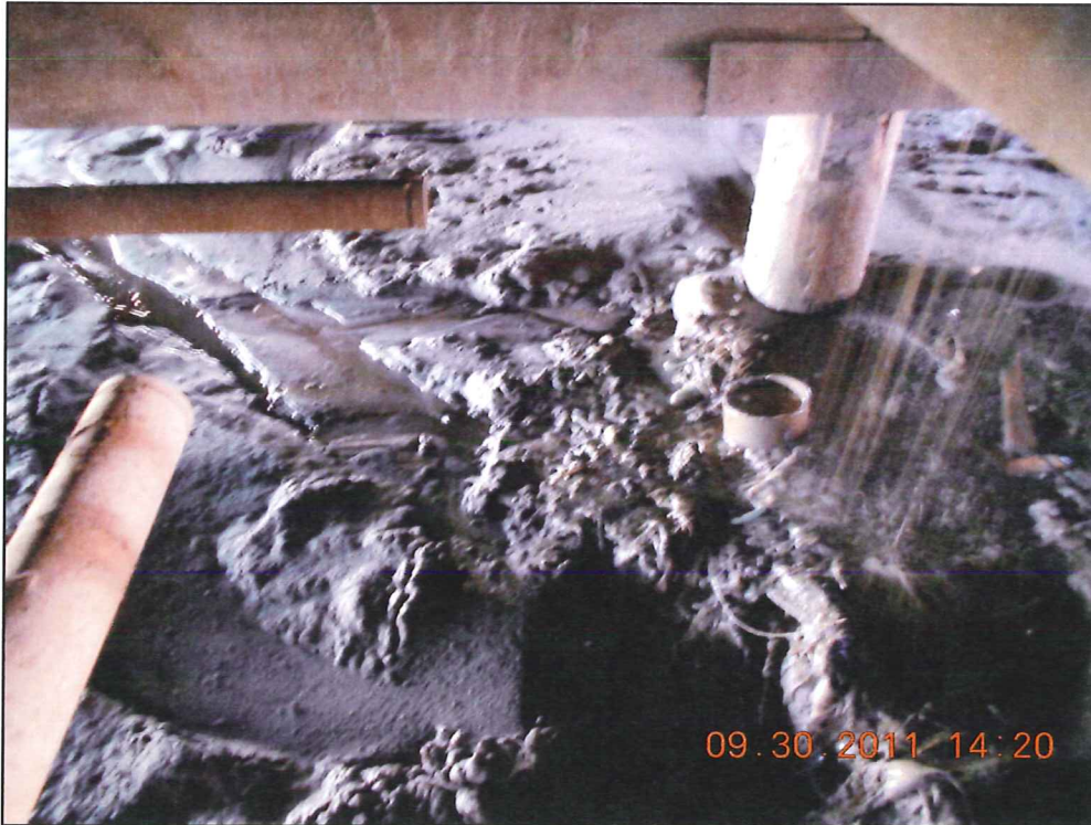
Water on right of photo pours through drain hole underneath building. Drain pipes shown disconnected.
