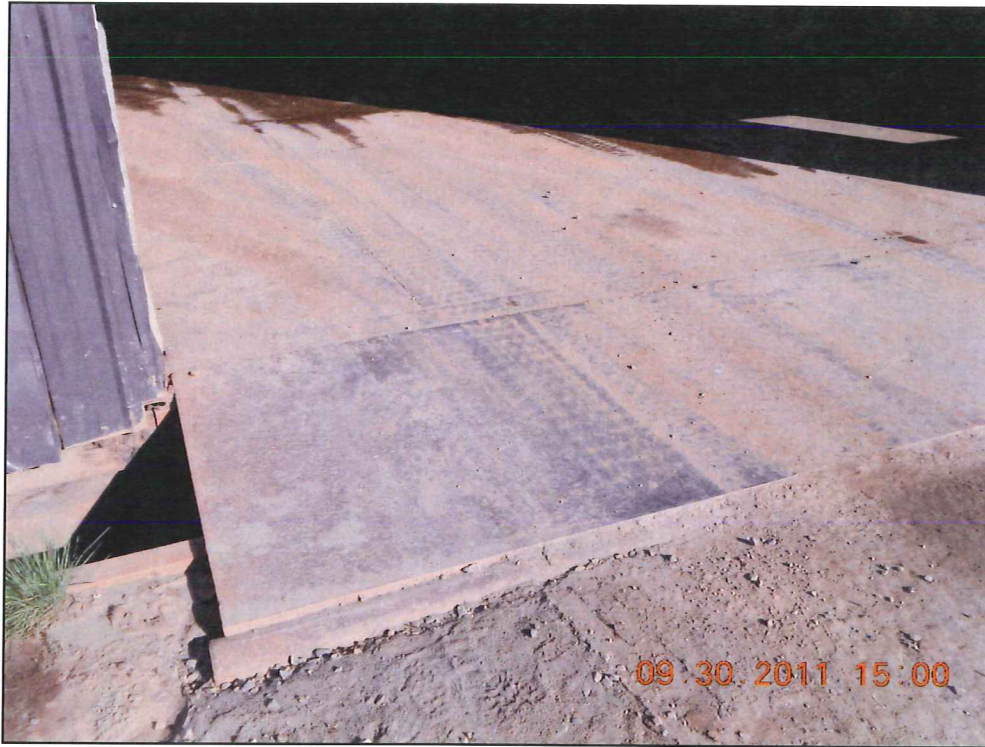
South ramp repaired in 2009 shows metal "bridge" for trucks to enter and exit garage. Wooden ramp was separated from contact with wet dirt as part of the fix.
