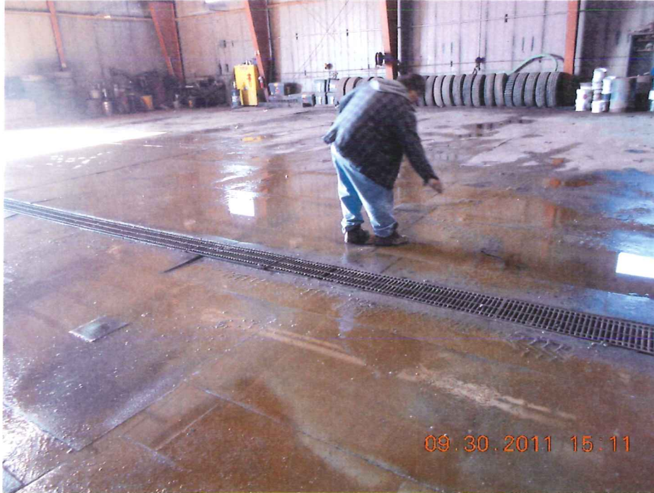
Property Maintenance Foreman Clair Grifka examines floor cracks. Floors wet from continuous use of pressure washer throughout the day to wash dirt off trucks.
