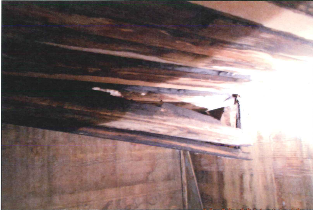
Several 2 x 8s visible under building— broken and falling down from rot.
