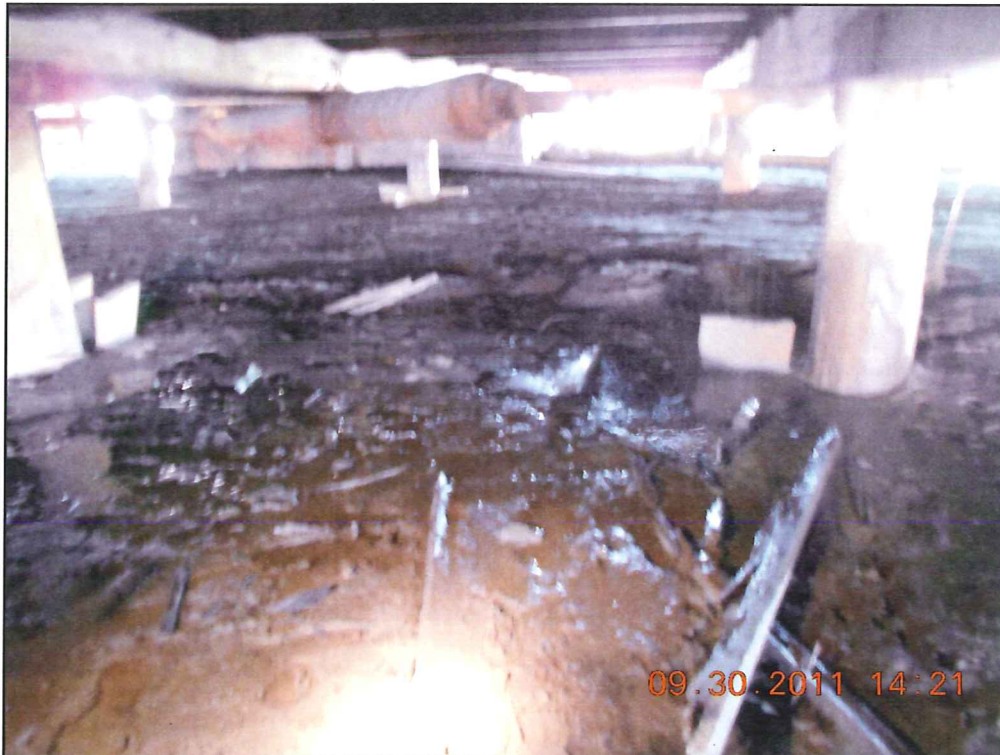
Sections of 2 x 8 floor supports shown on the ground after rotting and breaking off.
