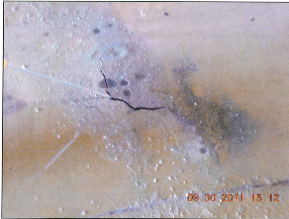
Crack several inches long in 3/16" thick metal sheets on City Shop floor.
