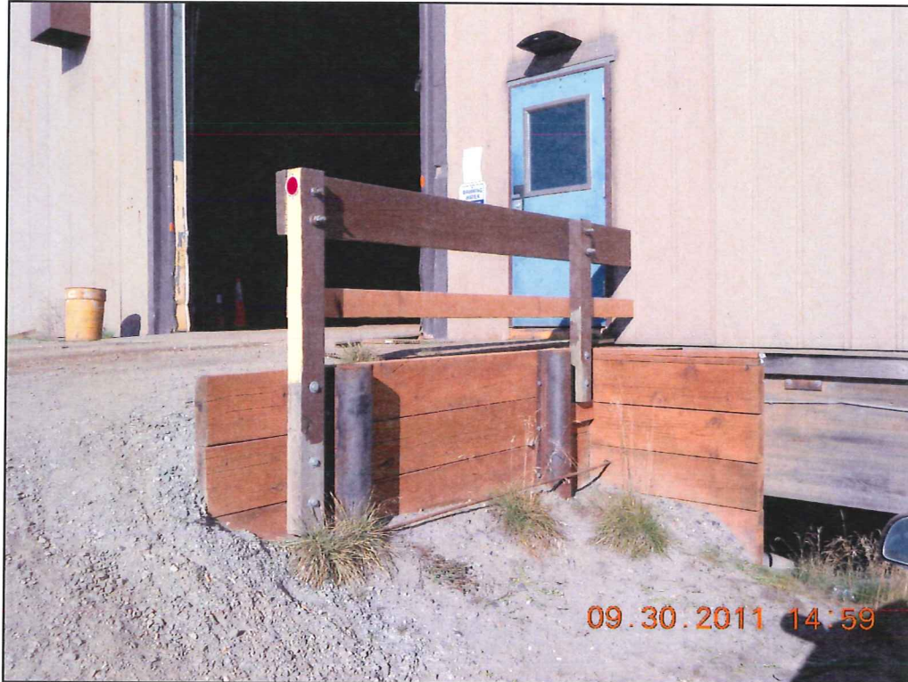
South ramp repair included construction of this bulkhead with treated wood to hold ramp dirt in place and separate ramp from building at the same time.
