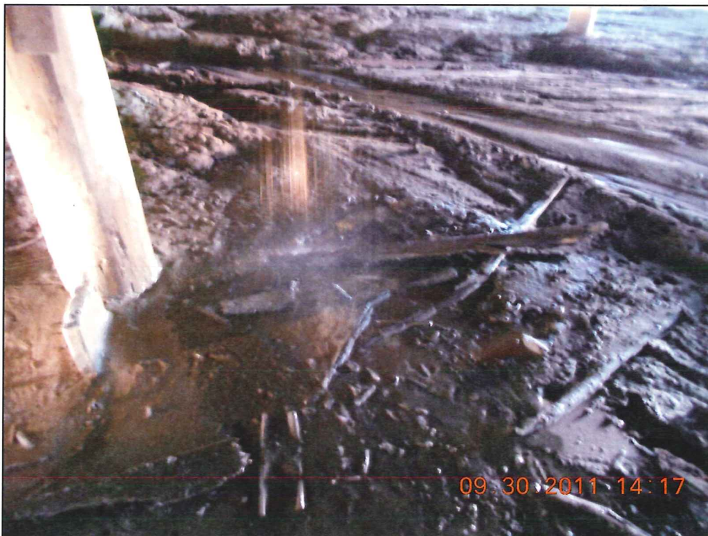
Water raining down through one of four drain holes contributing to rotting floor boards.
