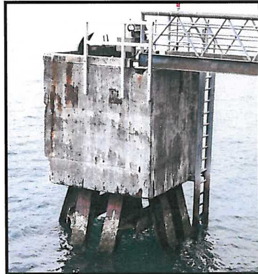
Figure 3: Condition of Existing Dolphin
