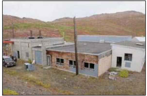
Launch Control Building, fall 2011 after volunteers replaced doors, shored up a sagging wall and began replacing the siding.
