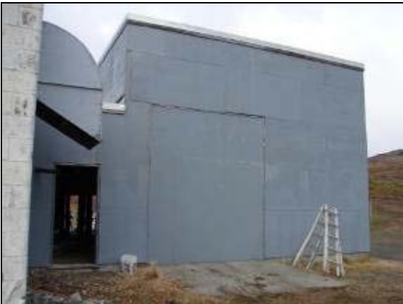
Volunteers installed a temporary plywood seal on one of the Launch Control Building doors to keep out vandals and the elements. This is one of the doors that needs replacing.
